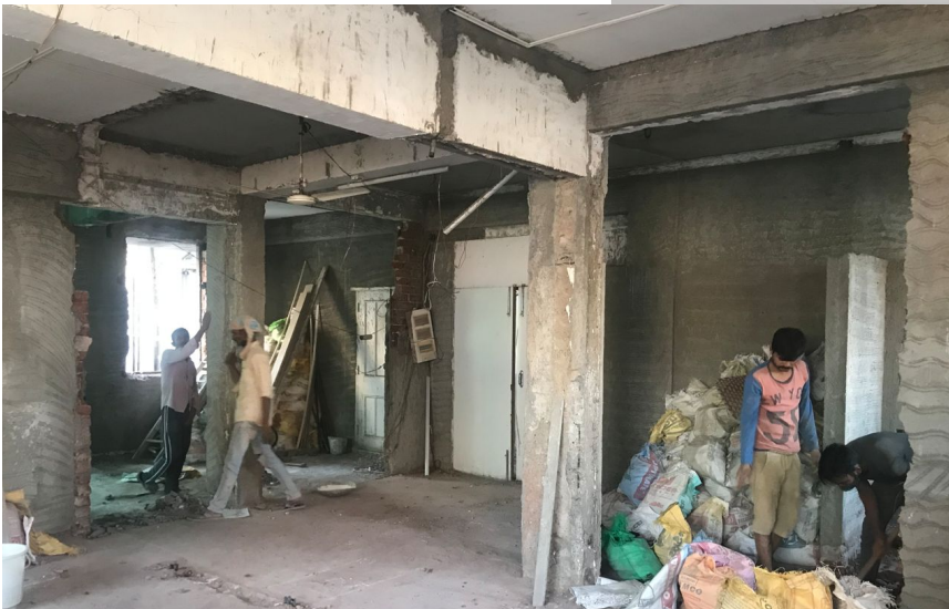
Existing Site Image
